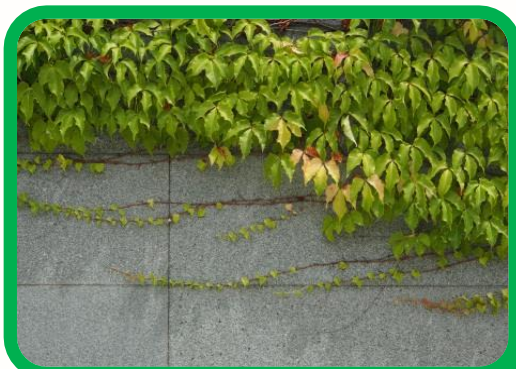
Wall covered by climbing plant
