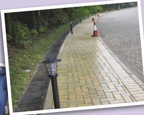
停車場的路旁安裝了10枝太陽能路燈 10 solar powered lights were installed to provide illumination for outdoor areas
